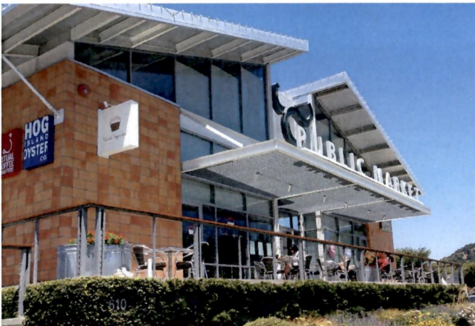
Use of trellis / awning to weather protection and to lend a pedestrian scale to street level
