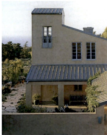
Stucco finish with metal roof
