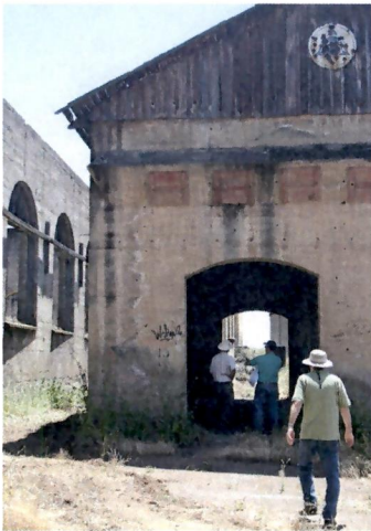
Ruins structures today
