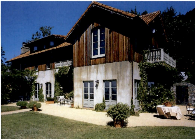
Appropriate use of accent material to create a signature architecture style
