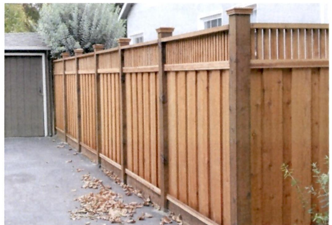
Traditional residential wood fence
